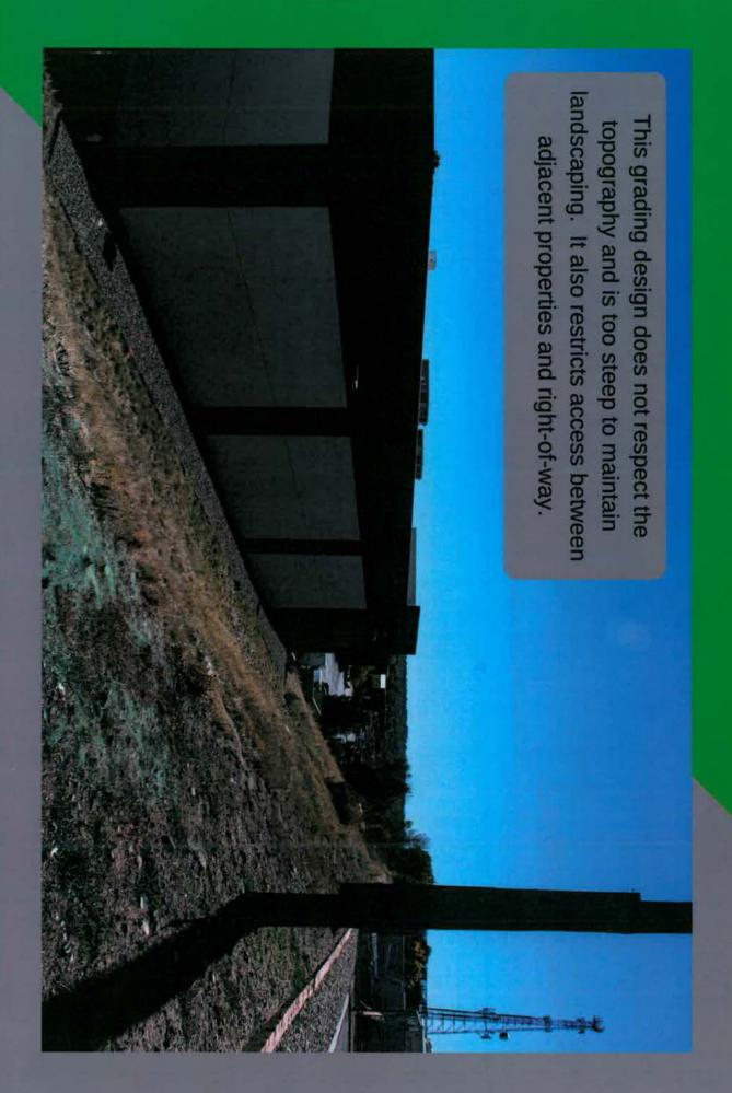
GRADING gr RETAINING WALLS This grading design does not respect the topography and is too steep to maintain landscaping.
