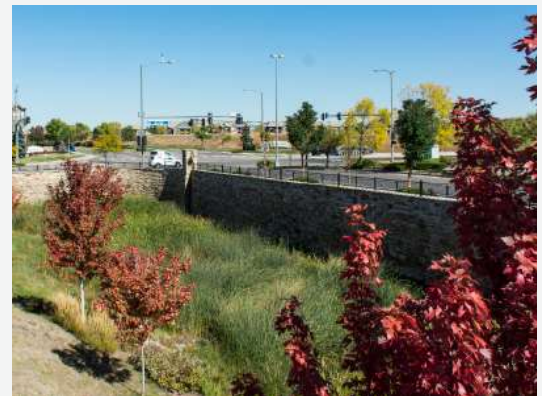
Stormwater Facilities. Trees, wetland plantings, and stone walls (natural or stamped) soften stormwater facilities that are visible from a public street.
