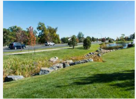
Stormwater Facilities. Rocks and wetland plantings make this drainage channel a visual amenity that complements the area.
