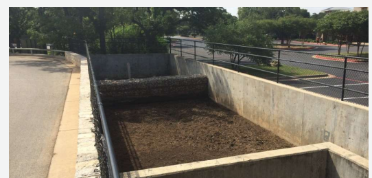
Stormwater Facilities. These two designs would NOT be permitted. Concrete structures and basins require rocks, landscaping, and/or surface treatments to soften their appearance.
